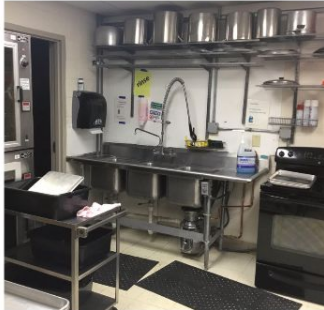
UNSAFE/UNDERSIZED SPECIAL ED SPACES
